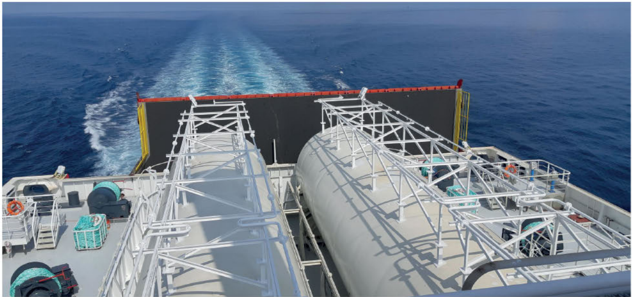
EACH TYPE C LNG TANK HAS A MAXIMUM CAPACITY OF 250M 3 WITH A 95% FILLING RATE LIMIT. SOURCE: CAPTAIN PHILIPPE SILLAN
